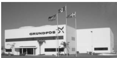
GMX - Monterrey, Mexico
